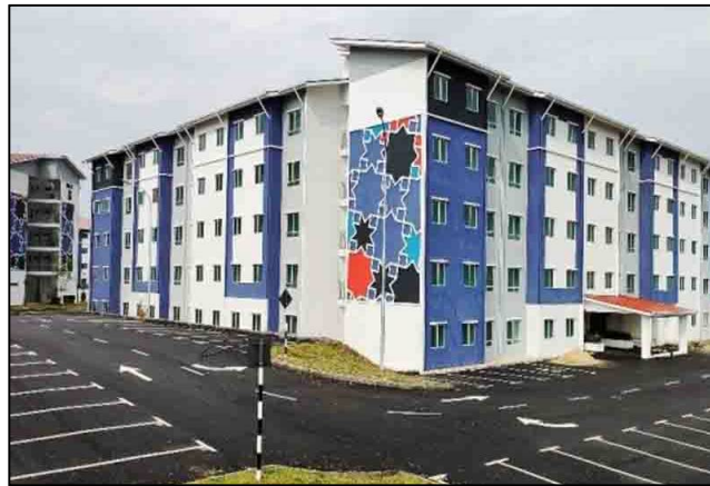
Figure 9: Flat Program Perumahan Rakyat (PPR), 418 units, 5 Storey Flat Machang PPR, Kelantan Darul Naim.
