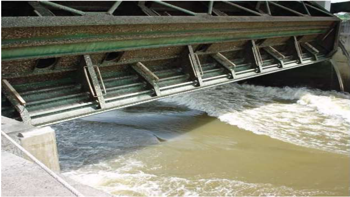
Figure 6: Barrage gate in open position
