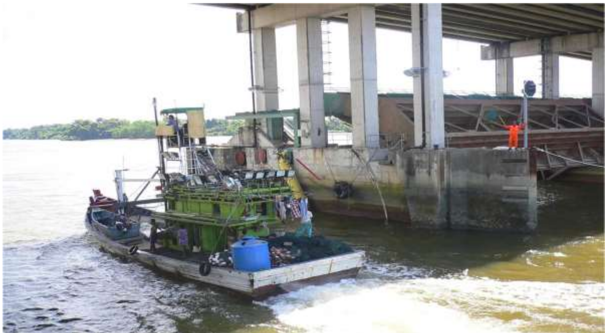
Figure 8: Barrage gates 4 and 5 in the open position with fishing vessel transiting gate 5 Risk aspects of the barrage
