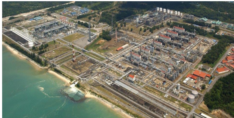
Figure 2: On-Shore Plant Facility
