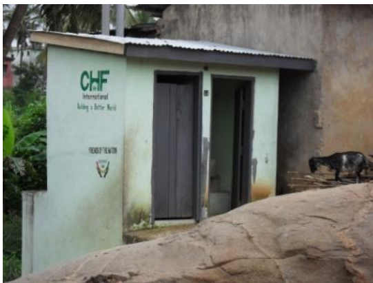
Fig. 3: A sample of Toilet Facility
