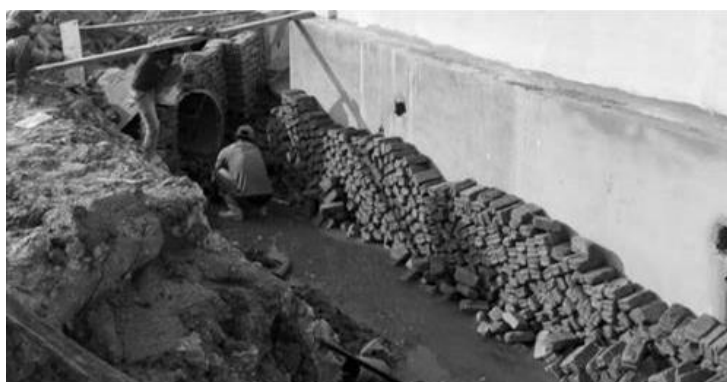
Figure 5. Workers rectifying a defect in the roadside drain.
