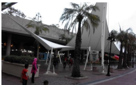
Figure 23: The unarrangement and design of tensile in the courtyard of the Souq that have less shading effect, messy and obstruct the view towards the Souq (Author, 2021).
