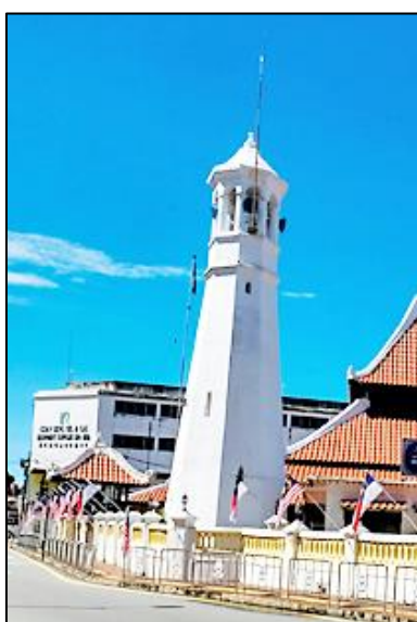
Figure 1.8: The Minaret of Masjid Kampung Hulu
