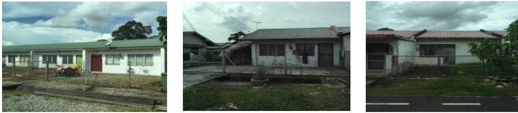
Figure 1: Examples of low-cost terrace houses
