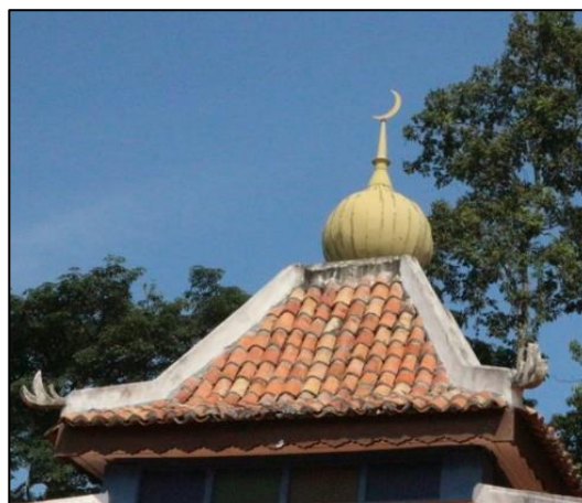
Figure 1.7: Roof Crown of Masjid Lama Machap
