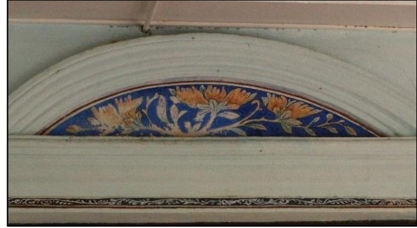
Figure 1.22: Decoration using chrysanthemum motif at the semi-circular arch panel Source: Field work
