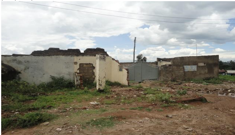
Plate 1. A Destroyed School in Lugari Sub-County
