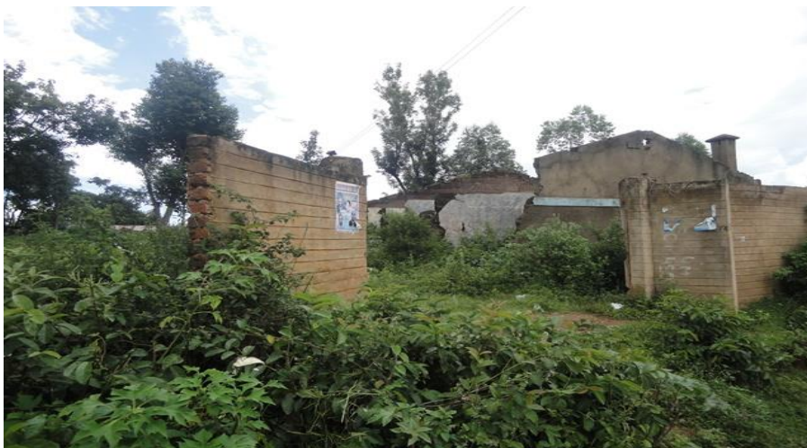
Plate 2 A Destroyed home in Kakamega Sub -county
