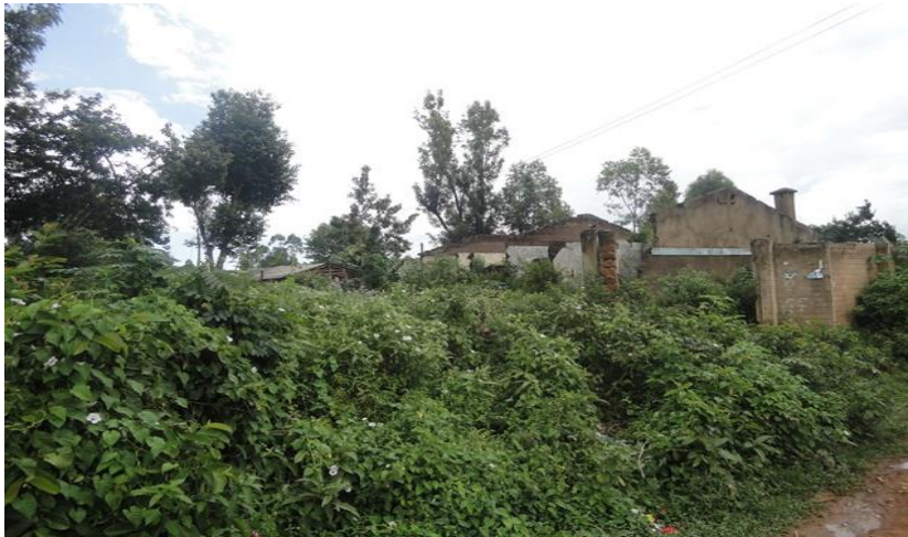
Plate 3 Destroyed home in Mumias Sub-County
