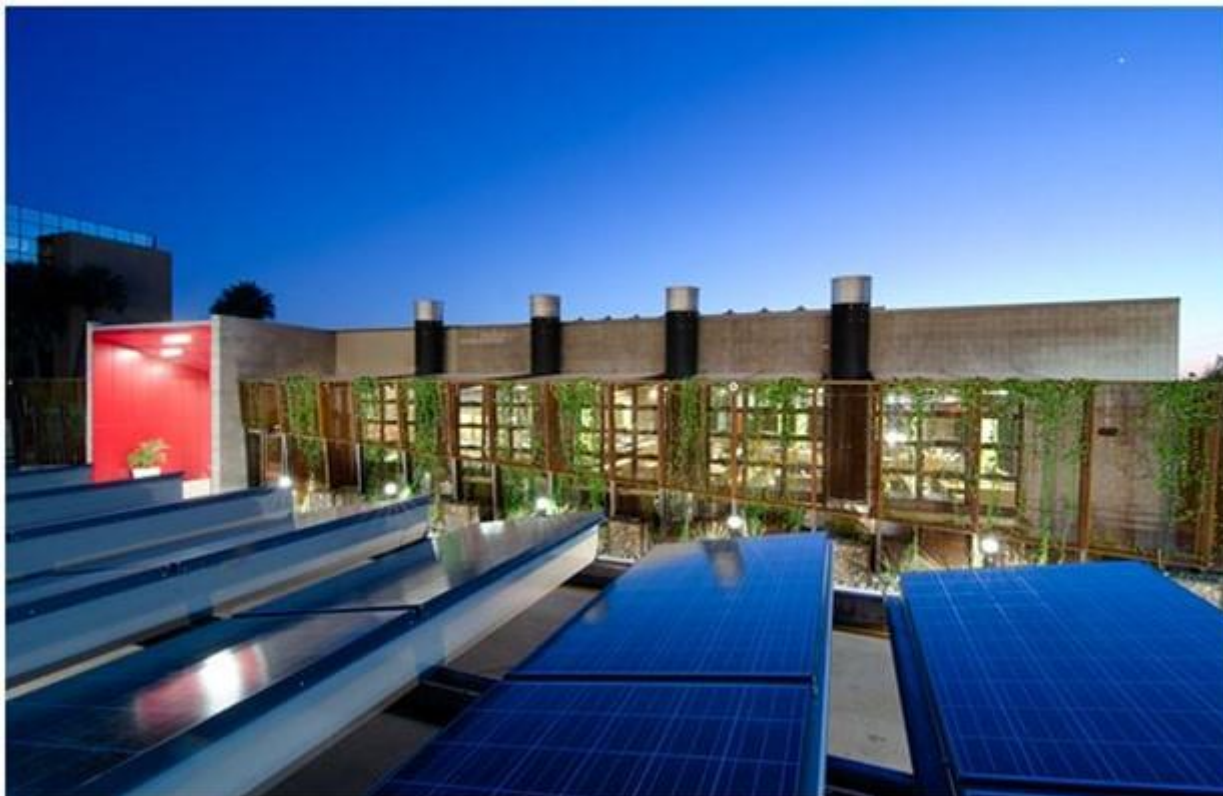
Figure 3: DPR Construction's Phoenix Regional Center, Arizona (image from DPR Construction Phoenix Regional Office | WBDG - Whole Building Design Guide, n.d.)
