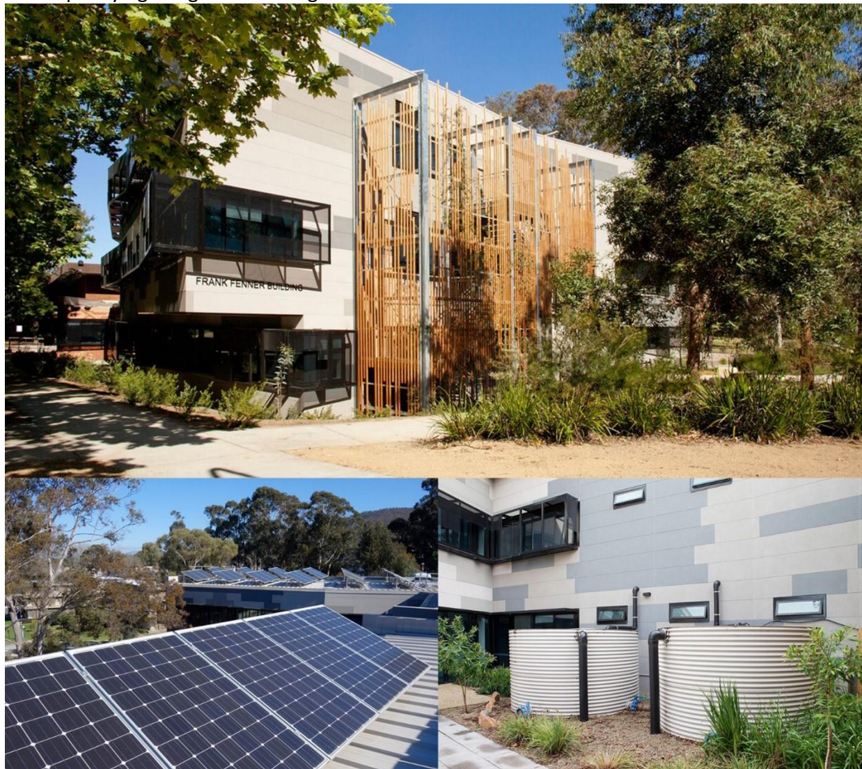
Figure 1: Frank Fenner Building, Fenner School of Environment and Society, ANU, showing views of solar panels on roof and the water recycling system (Australian National University, n.d.).
