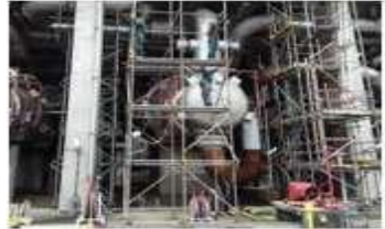
Erection of scaffold more than 5m height for paint job
