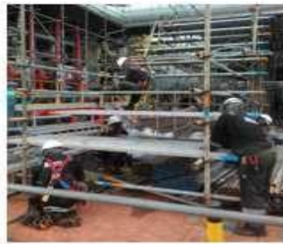
Erection of scaffolding as temporary platform
