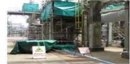
Hot work activity at height
