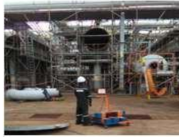
Manual handling to move material/equipment at site
