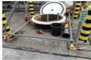
Confined space activity to do inspection work
