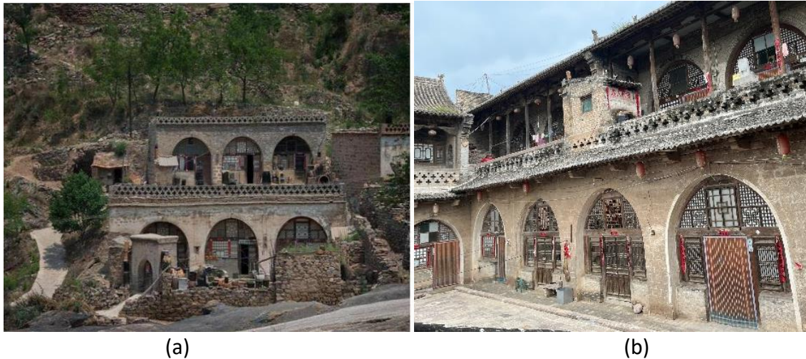
Figure 2. Architectural drawing of Shanxi cave dwelling. (a) Cliff-like cave dwelling; (b) Independent cave dwelling.
