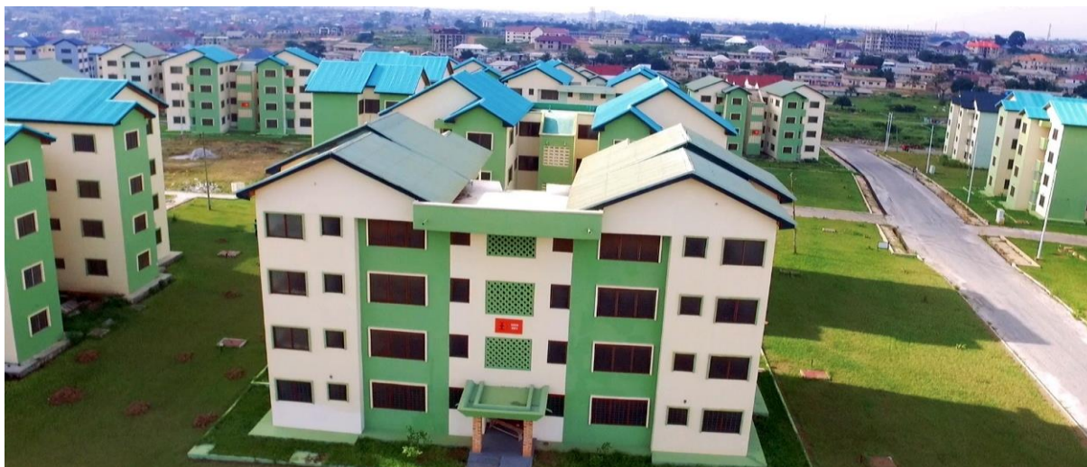
Figure 5. Completed Asokore-Mampong Housing Project
