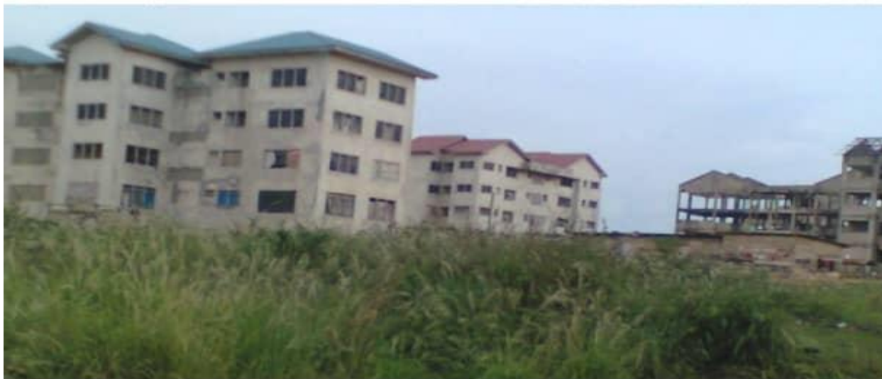
Figure 3. Asokore-Mampong Affordable Housing Project Abandoned in 2009 Source: Twumasi-Ampofo et al (2014)
