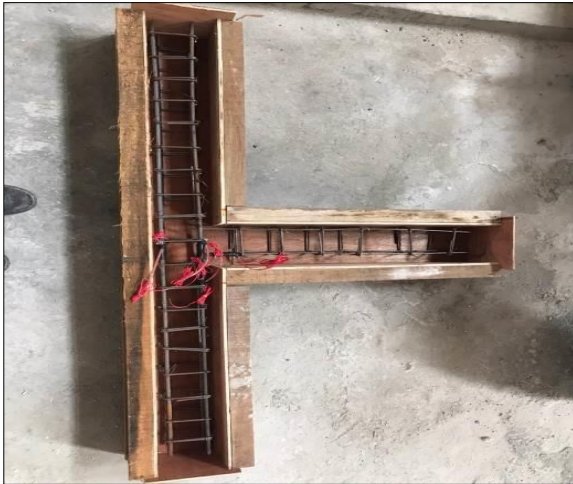
(a) Installing Reinforcement Bars in The Formwork
