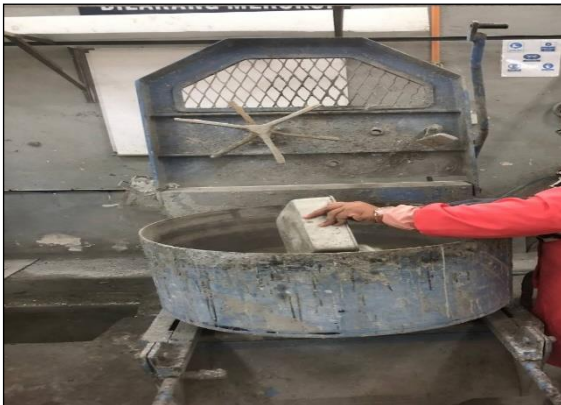
(i) Mix for R-ECC Using Concrete Mixer Pan
