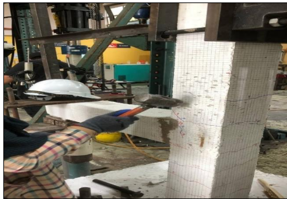
(c) Roughness The Surface Using a Sledgehammer
