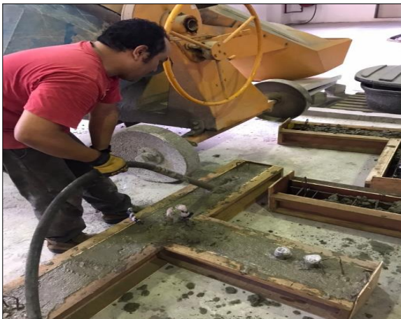
(c) Vibrating Concrete Process
