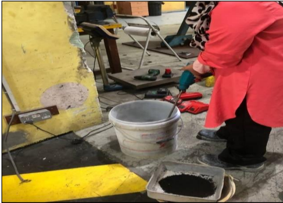
(g) Mix for Base Lining Using Concrete Mixer
