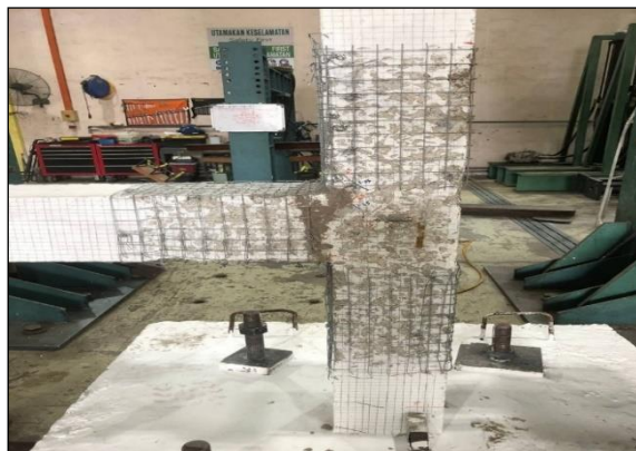
(e) Installing Wire Mesh
