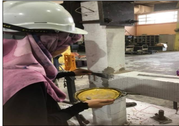
(b) Repairing The Crack Area Using Concrete Seal
