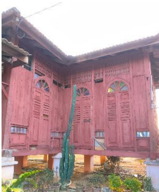
Figure 2 Traditional houses usually have perforated carvings ( ukiran tebuk tembus ) above doors and windows to allow better natural light and ventilation inside the house.
