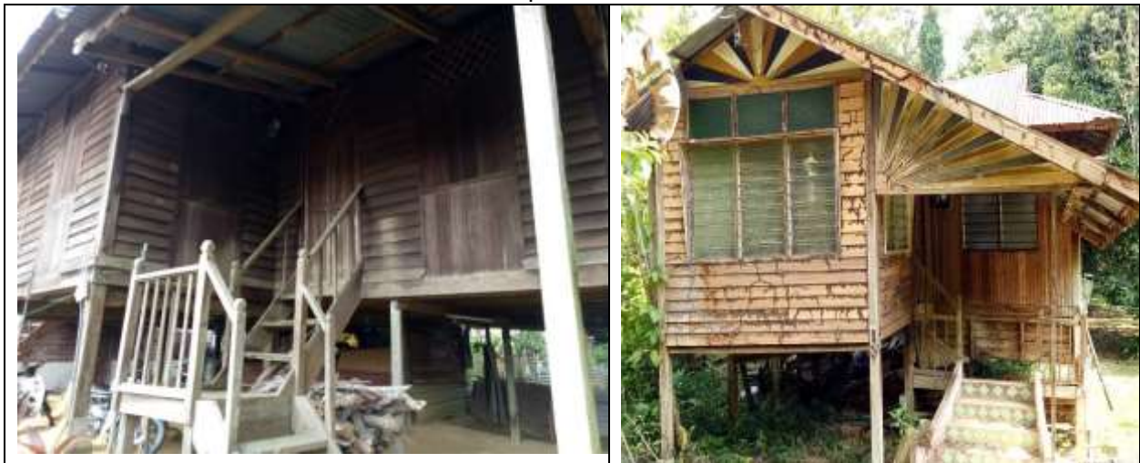
Photo 7. The traditional houses that are not well-preserved.
