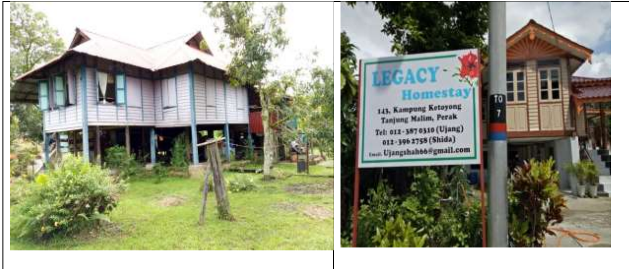
Photo 4. The Perak traditional Malay houses discovered during fieldwork.
