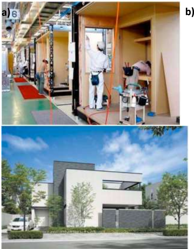
Figure 2 (a) Toyota Home Module fabrication at Toyota Home factory in Japan (b) Rendering of one of Toyota customizable home designs adopted from (Abulfahem, 2012)
