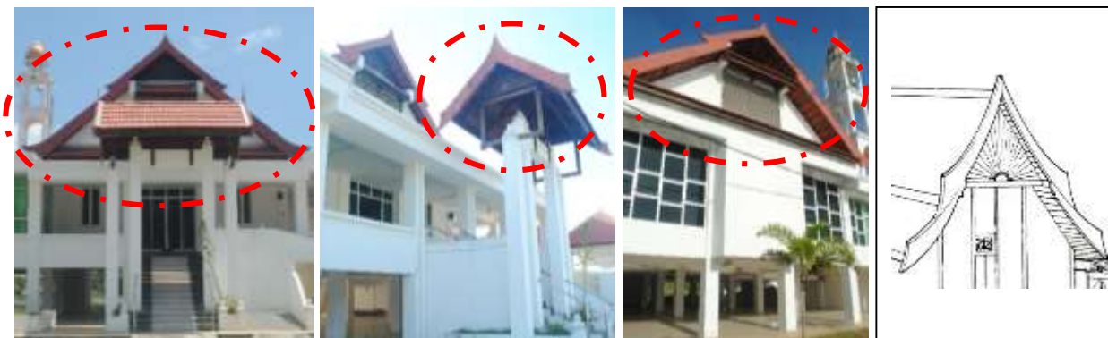
Figure 4. The Image of Pemeleh for Mukim Masjid Mosque, Kota Bharu. Source: Norhidayah, (2016).
