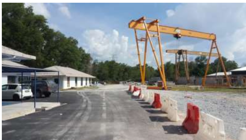
Figure 3: The offsite prefabrication factory facilities (Courtesy: Company B)
