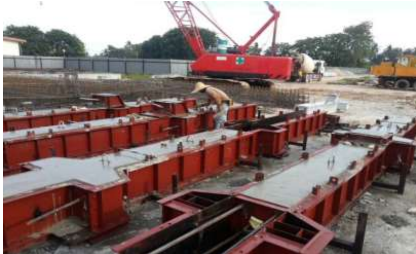
Figure 2: The onsite prefabrication yard (Courtesy: Company A)
