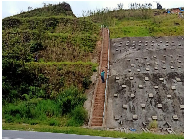
Figure 2. Photo of the site on October 2020
